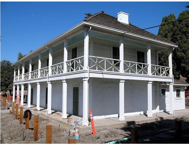
Alviso Adobe undergoing renovations last fall
