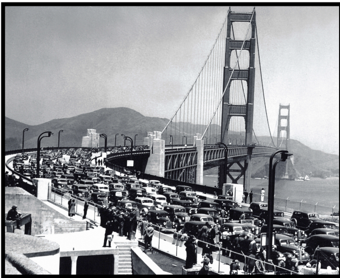
The Golden Gate Bridge on Opening Day, May 27 th , 1937
