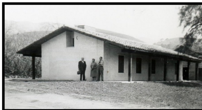
After the Higuera Adobe was restored.
